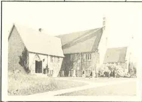
FOREST HILL UNITED CHURCH (Erected 1940) Bathurst Street and Wembley
