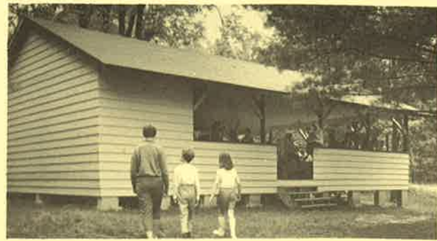
CRAFT HOUSE: Newest building in camp and a very popular spot for those activities where campers use their hands to make things.
